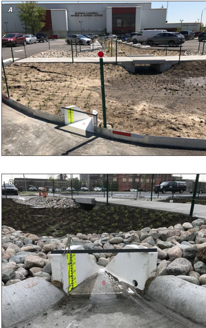
Figure 21. Photographs showing A , the metal border between the parking surface and rain garden and an H-flume used to measure runoff at Gary City Hall in Gary, Indiana, and B , the H-flume used during the study. Photographs by David C. Lampe, U.S. Geological Survey.
