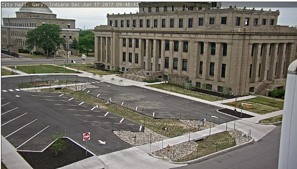
Figure 3. Gary City Hall in Gary, Indiana, after construction of the green infrastructure and rain garden (2017). Massachusetts Street in the foreground. Photograph by the U.S. Geological Survey.
