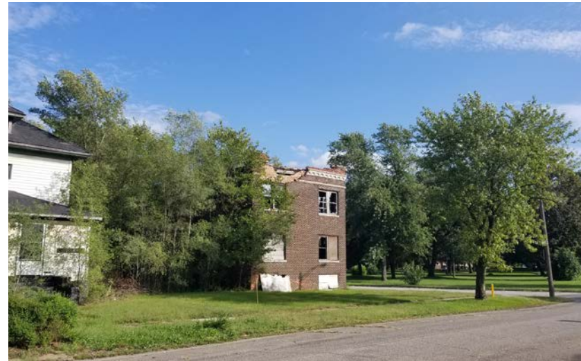
Abandoned buildings across from Buffington Park in Emerson provide an opportunity for a number of potential uses
