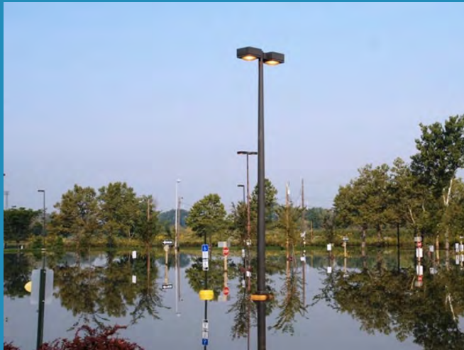
Flooding at Indiana University Northwest north parking lot (2008)
